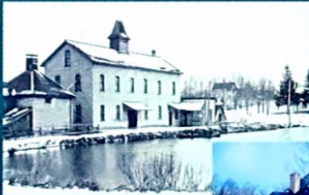
ABOVE AND RIGHT: The oat mill on Mill Street was one of the largest buildings in town. It was built in 1886 and was demolished in 1957 after part of it collapsed. The small building beside it was the kiln for drying the grain, and it is still there (photo on right), used as a residence.
