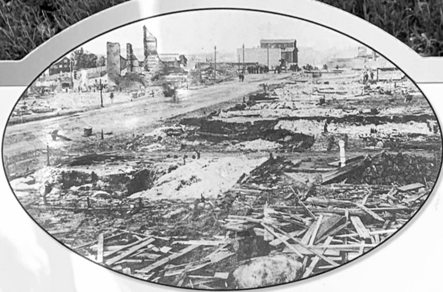
The morning after the fire in downtown Port Perry, 1884. The Grain Elevator can be seen in the background, having survived the devastation.
