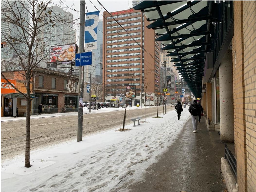
Figure 19: Example awning on Dundas St, looking west from Church. Ideally, the awning would be wider and longer than this.
