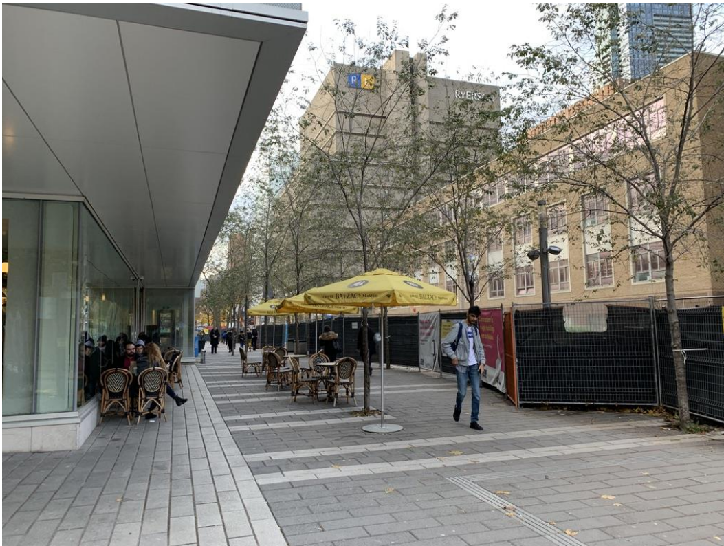
Figure 17: Construction ironically creates a quiet atmosphere. The café was popular and the sidewalks were busy. Gould St & Bond St, looking west.
